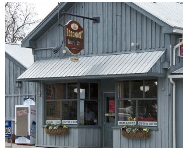
Board and batten exterior
