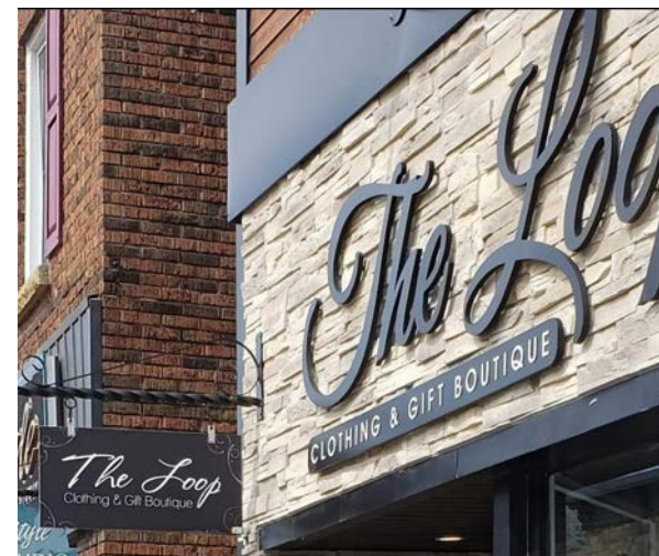
Stone veneer facade
