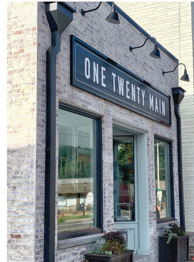
Column details with exposed brick, lighting, and signage
