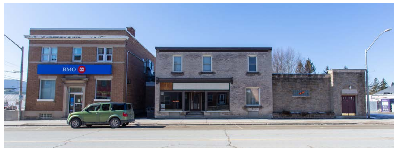
Yonge Street North - West Side (North of Matilda Street)
