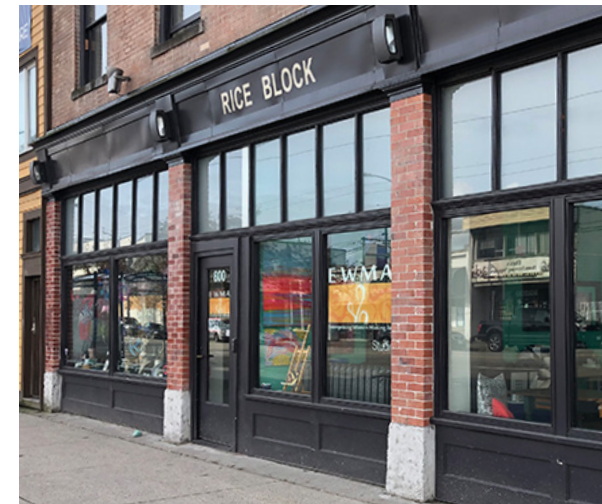
Painted transom and window details with exposed brick columns
