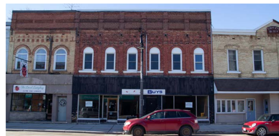
Existing Façade, February 2023
