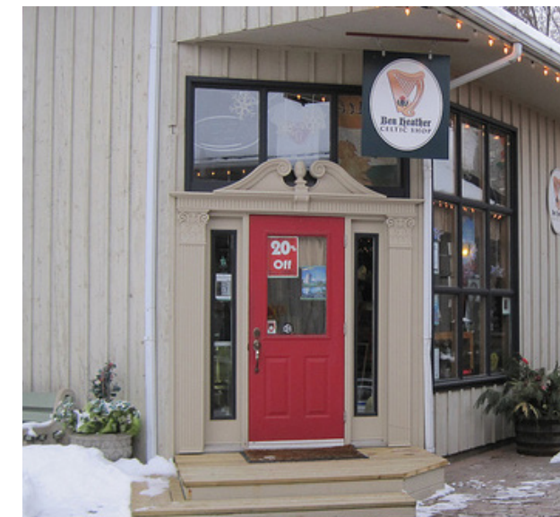
Board and batten exterior
