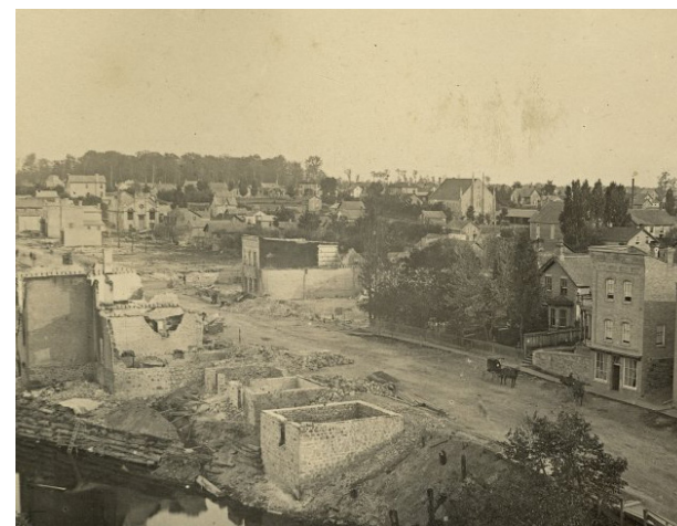
Few Main Street Buildings Remained After The Fire In 1888
