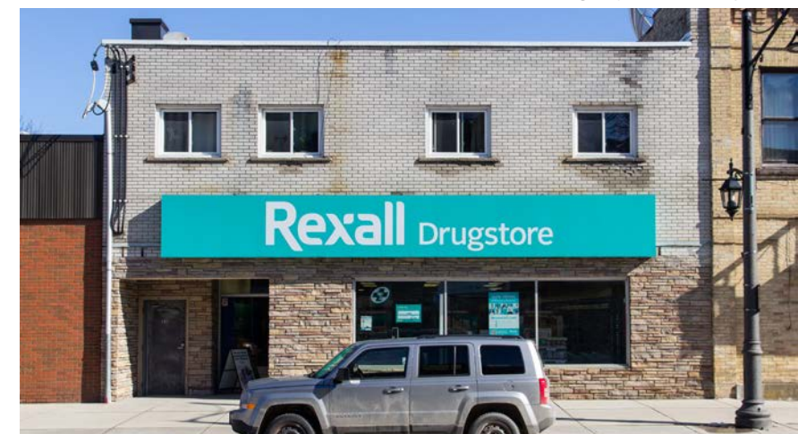
Existing Façade, February 2023
