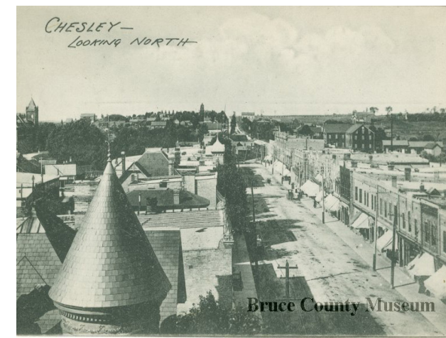
View of Main Street Looking North, 1908
