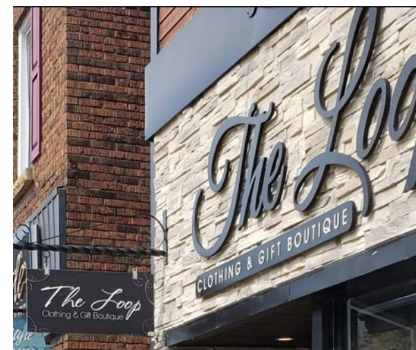
Stone veneer facade
